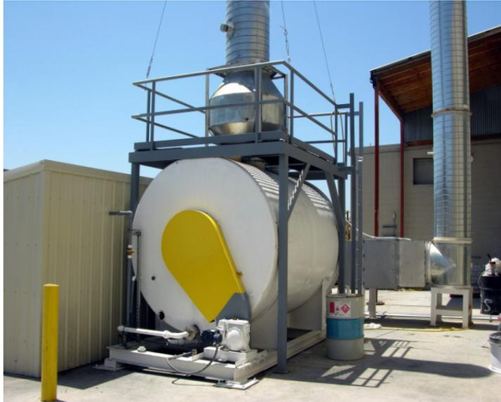
***The Filtercrobe system is able to eliminate the Hydrogen Sulfide, Siloxane, Thiols (Mercaptans) and Nitrogen compound by least 98%. Guaranteeing pure processed methane providing endless benefits to the owner/operator including reduced processing increased maintenance intervals and longer equipment life.***
